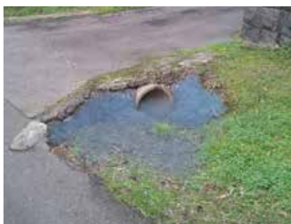
Use for pooling water anywhere.
