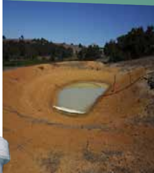
Leaking dam walls
